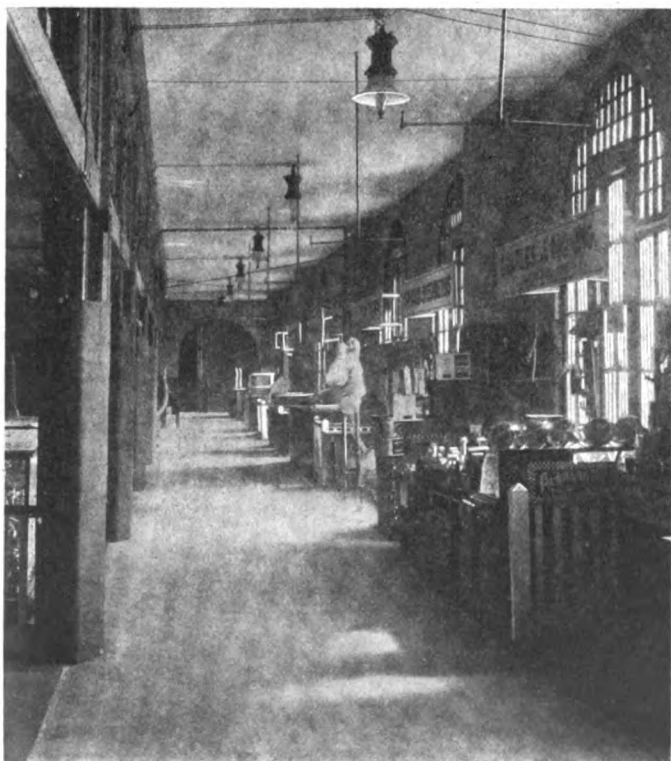
An Aisle in the West End of the Main Building.
